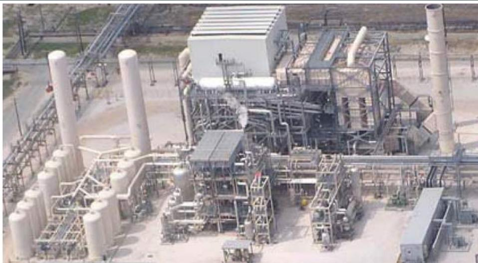
Methane steam reforming for H<sub>2</sub> production (112,000 Nm<sup>3</sup>/h)
